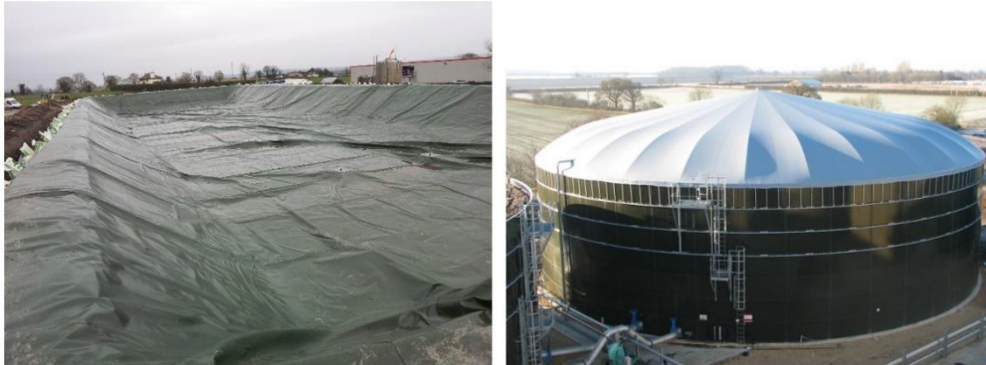
Figure 30 - Closed digestate storage - (left) covered lagoon, (right) sealed tank (source: Geoline 6 , Permastore 7 )
