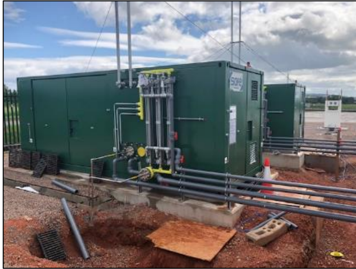
Compressor during installation
