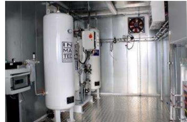
Figure: example O_2 generation system
