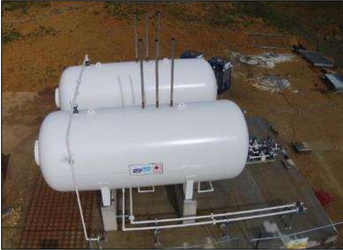
Mounded Propane Storage Cumbernauld - 1 x 12 tonnes
