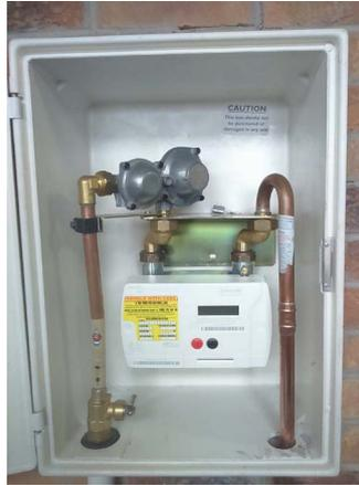
Figure 24: Recessed Meter Box Internals
