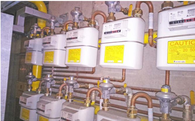
**Figure 40:** Purpose-built meter manifold
