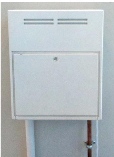
**Figure 14** Surfaced Mounted Type Meter box
