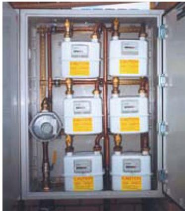
**Figure 25:** Pre-fabricated meter cabinet
