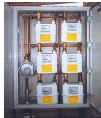
**Figure 34:** Pre-fabricated meter cabinet
