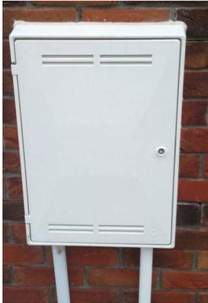
Figure 23: Recess Meter box
