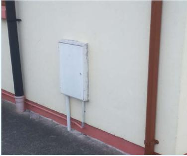
At the front gable end wall, a maximum of 2 metres from the front corner of the building. Fig 8.
