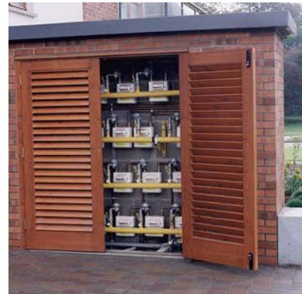
**Figure 41:** Purpose built meter manifold in purpose built meter compartment block/brick construction
