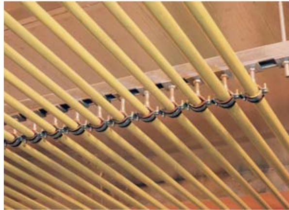
**Figure 33:** Supply pipework supported at ceiling level
