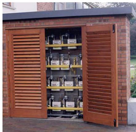
Figure 26: Purpose-built meter manifold
