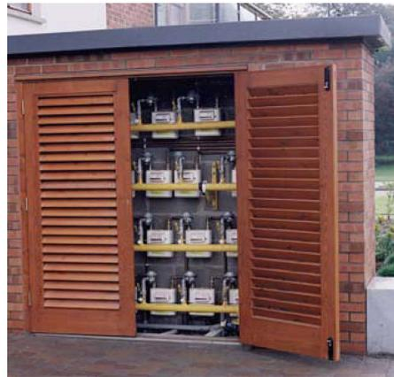
**Figure 26:** Purpose-built meter manifold
