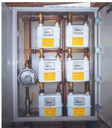
Figure 25: Pre-fabricated meter cabinet
