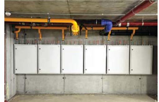
Figure 29: Top entry cabinet pre-fabricated off site.
