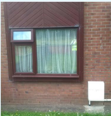
At the front wall of the building – on either side of the front door, or on either side of a sealed window. **Note:** This can't be fitted directly below a window.
