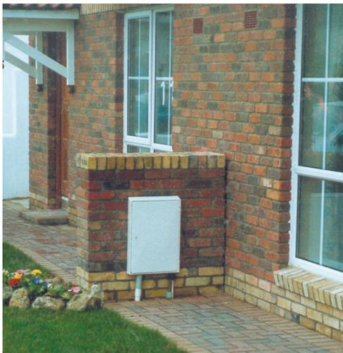
Figure 20 Meter box in pillar enclosure
