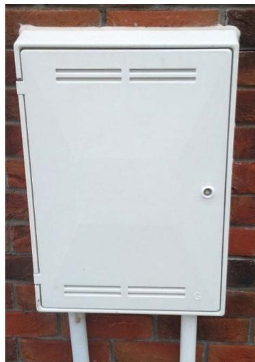
**Figure 15** Recessed Type Meter Box
