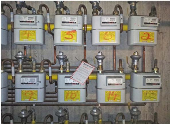
**Figure 32:** On-site meter manifold
