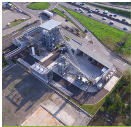
Figure 3 Gasification production process. Source: ENGIE
