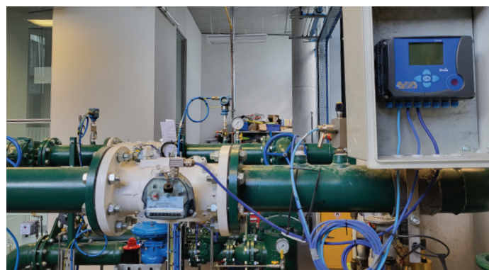
Figure 3. Volume corrector typical install
