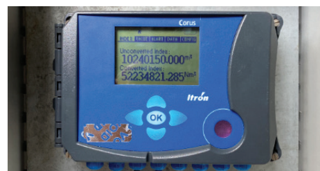
Figure 5. Volume corrector (unconverted and converted index screen)
