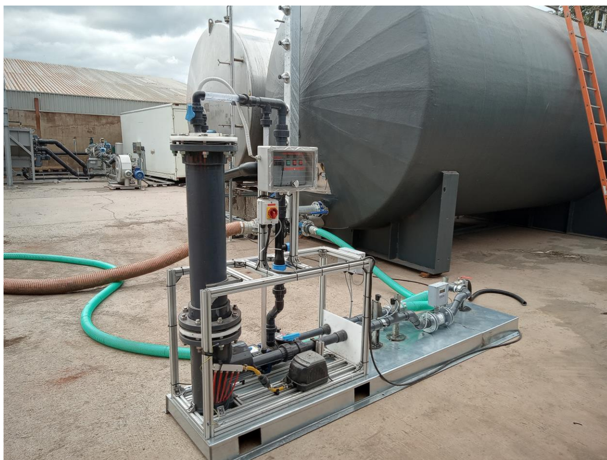
Fig. 4: On-site installation at a UK digestate facility of large-scale unit
