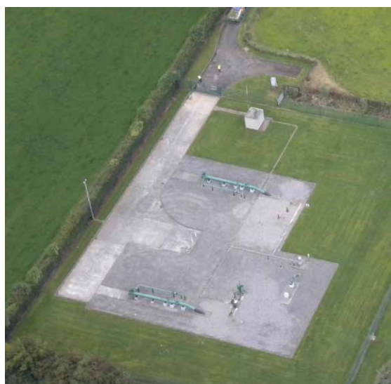
Figure 10.2 Aerial View of an AGI Site
