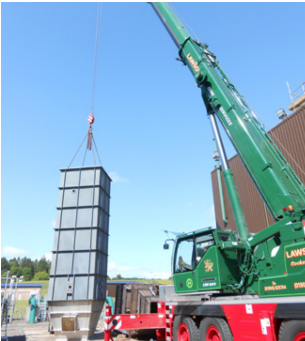
Figure 10.2: Vent Stack Replacement at Beattock Compressor Station
