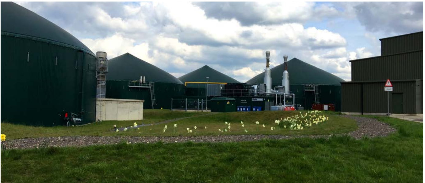
Figure 6-2: Agrivert anaerobic digestion facility, Wallingford, UK
