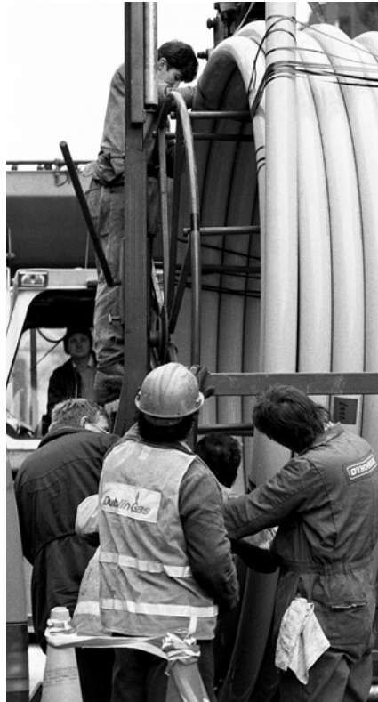
Dublin Gas Construction 1990
