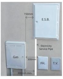
Minimum separation from recessed gas meter box to the electricity meter
