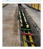
**Open Cut** – installing pipe using standard trenching techniques. Pipe is laid with a sand or pea gravel surround and gas marker tape is laid above the sand.
