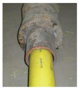
Insertion – utilising existing metal gas mains / services as a carrier for new PE pipes. Inserted PE may be a close or loose fit. The carrier pipe is broken out at connection points, i.e. at pipe joints or where a gas service pipe is connected.
