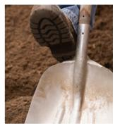
Hand digging using shovels and spades presents the lowest risk of damaging a gas pipe.
