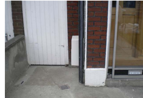
Gas Networks Ireland reinstatement.
