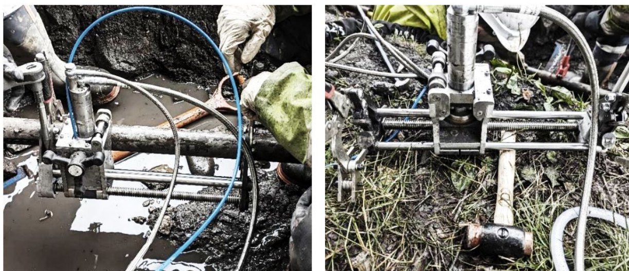
Figure 1-3:Service Connection using SWC.
