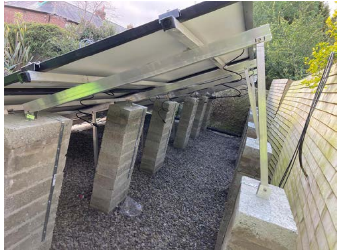
Picture 4: Blockwork supports for the solar panel array
