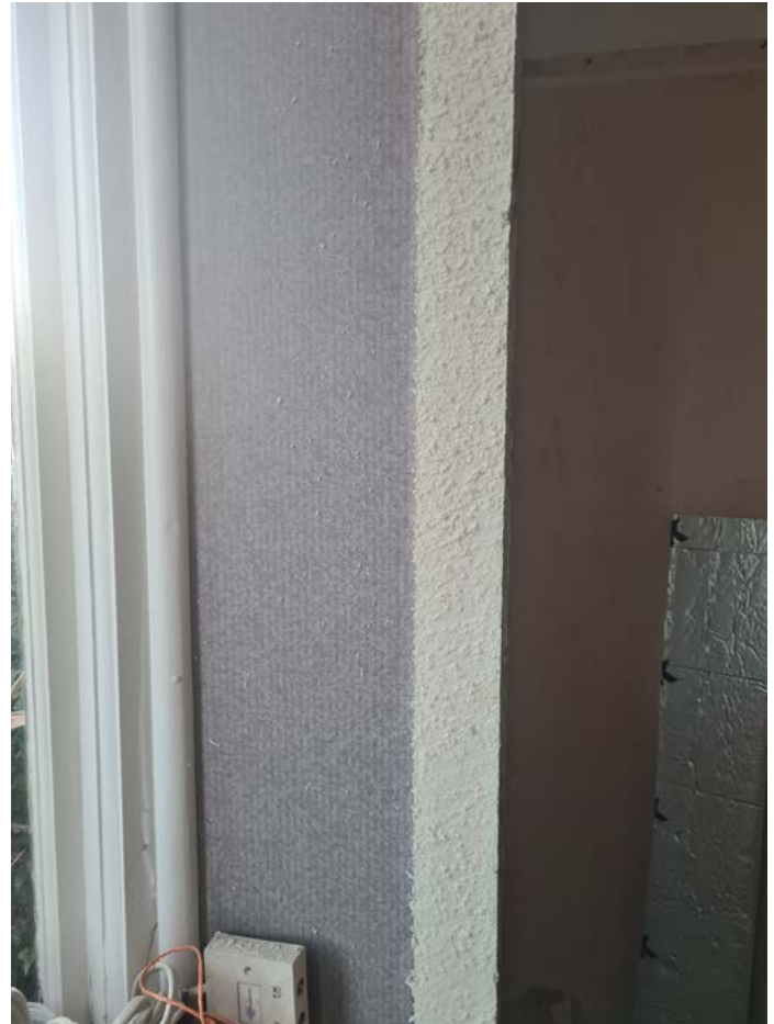
Picture 2: Internal insulation fitted tightly to the external wall including the window jambs, to prevent thermal looping occurring behind the insulation
