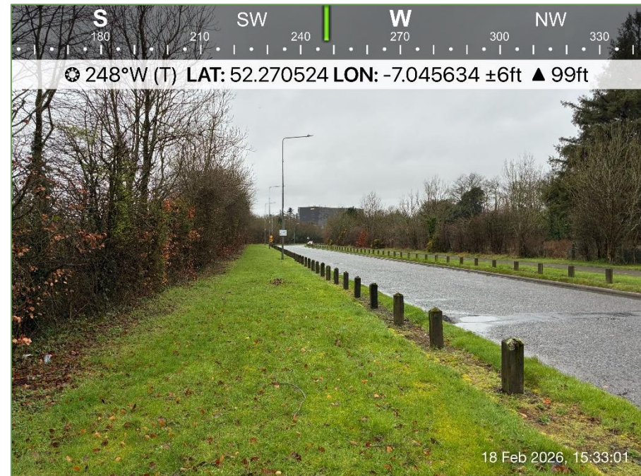
A4. View of the L3421 towards the Belview Science & Technology Park along which the proposed pipeline will be installed.
