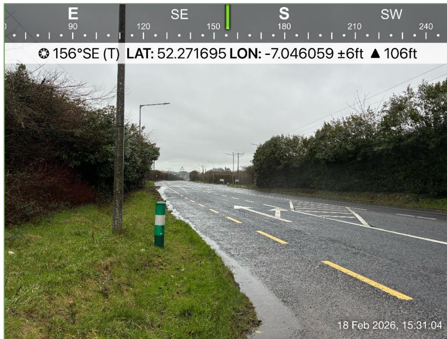
A3. View along the N29 leading along which the pipeline will be installed.
