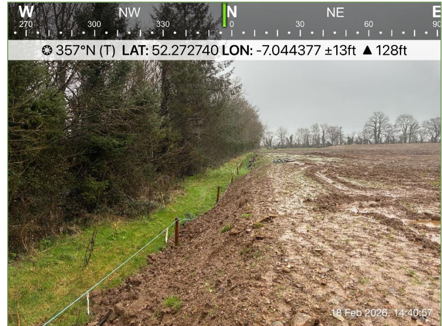
A2. View of the greenfield site currently under construction within which the pipeline will be installed.
