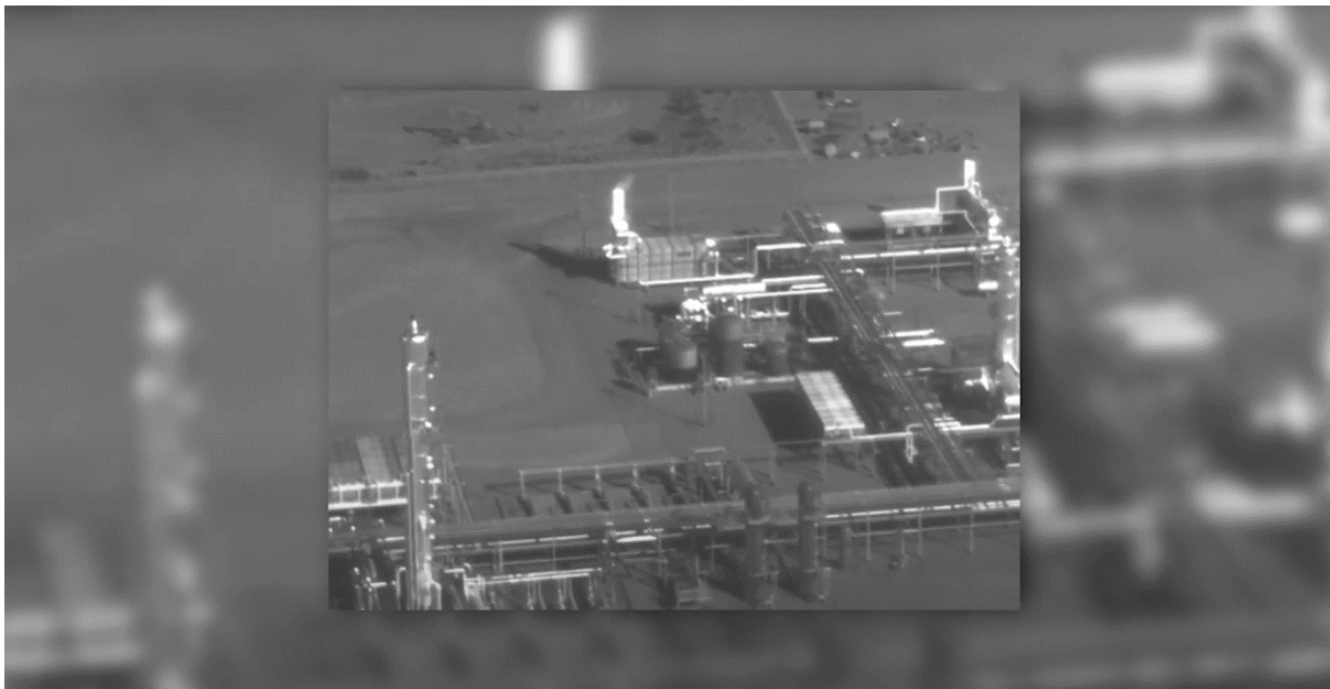
Figure 3 OGI thermal image showing methane plume visualisation at a gas facility [27].
