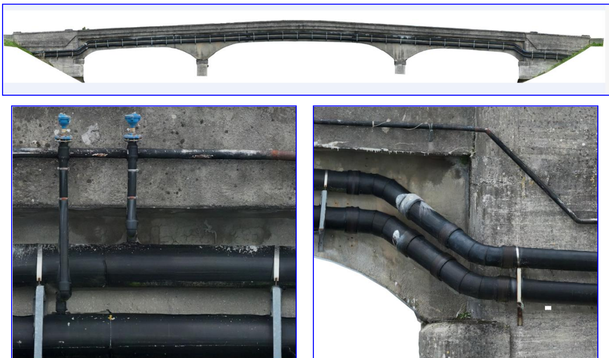
Figure 7 UAV close-range imagery of Ardnacrusha bridge gas pipeline crossing, Co. Clare, side-view orthomosaic (top) with detail views of pipe supports and fittings at bridge piers (bottom). Source: SurveyLabs Ireland [54]
