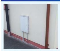
At the front gable end wall, a maximum of 2 metres from the front corner of the building. Fig 8.
