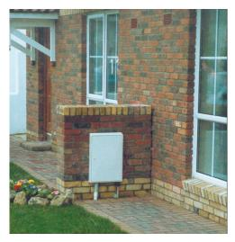
Figure 20 Meter box in pillar enclosure
