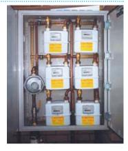
**Figure 34:** Pre-fabricated meter cabinet
