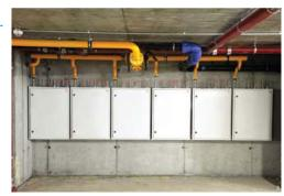
Figure 29: Top entry cabinet pre-fabricated off site.
