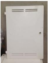
Figure 18: Recessed type meter boxes with vents
