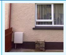
At the front wall of the building – on either side of the front door, or on either side of a sealed window. Fig 9.
