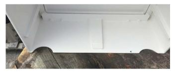
Figure 16: New cut outs at outlet pipe and inlet pipe
