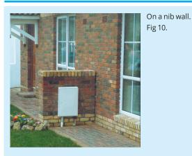
Figure 10 Meter box on nib wall
