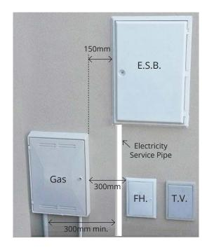
Figure 5 Minimum separation between Gas and other meters
