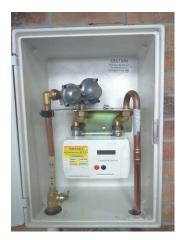
Figure 24: Recessed Meter Box Internals
