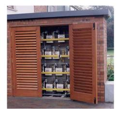
Figure 26: Purpose-built meter manifold
