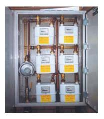
Figure 25: Pre-fabricated meter cabinet
