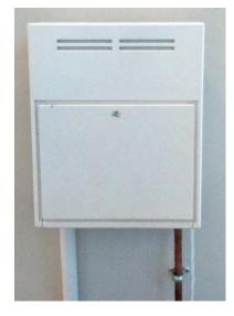
Figure 14 Surfaced Mounted Type Meter box
