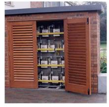
**Figure 41:** Purpose built meter manifold in purpose built meter compartment block/brick construction
