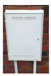
Figure 23: Recess Meter box
