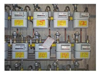
Figure 32: On-site meter manifold
